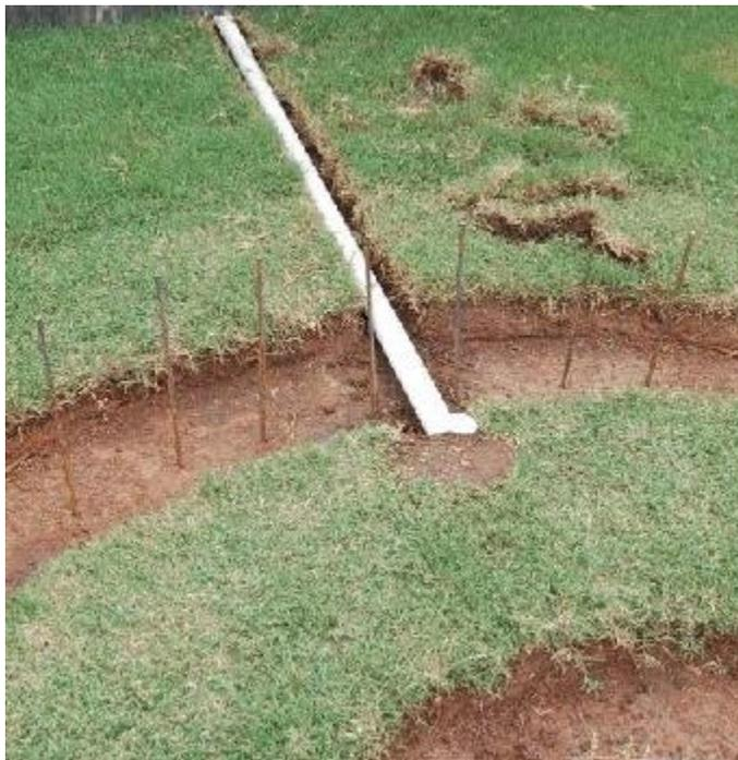
Step 5 → I decided to create a concrete base for under my Gas ring so I extended out the PVC pipe to reach to the Pit, and then I put in another drain.
