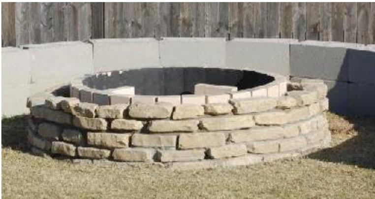
Step 15 → I finished the stone work and then poured mortar in between the fire brick and the stone for extra stability. Then I laid out the flagstone in the yard and tried to piece together this very difficult puzzle. Getting them to fit, in a circular pattern was not easy and it took about 2 hours to get a design that I was comfortable with. Once complete, I topped off the pit with more lava rock and then cleaned the stone and flagstone.
