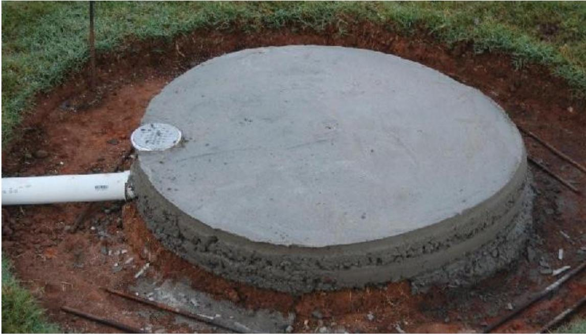
Step 8 → A trench was dug to run the gas line from the Propane tank to the fire pit. I dug down about 8 inches and placed 2" PVC pipe in the ground.
