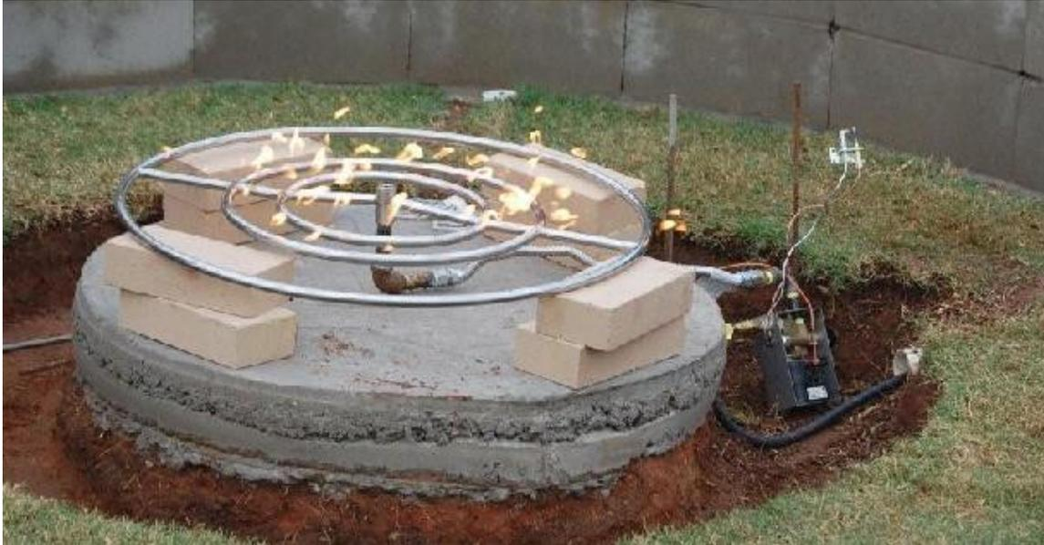
Step 13 → The footing for the fire brick and stone was poured and then the fire brick were put in. First a row of horizontal bricks and then the soldiers (vertical brick) were put into place to form a circle.
