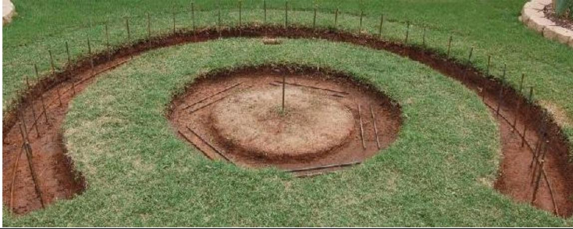
Step 4 → I wanted a drain for the sitting area because I didn't want water to gather at the back, where someone's feet would be. I created a slight slope so the water would drain through the PVC and under my fence.
