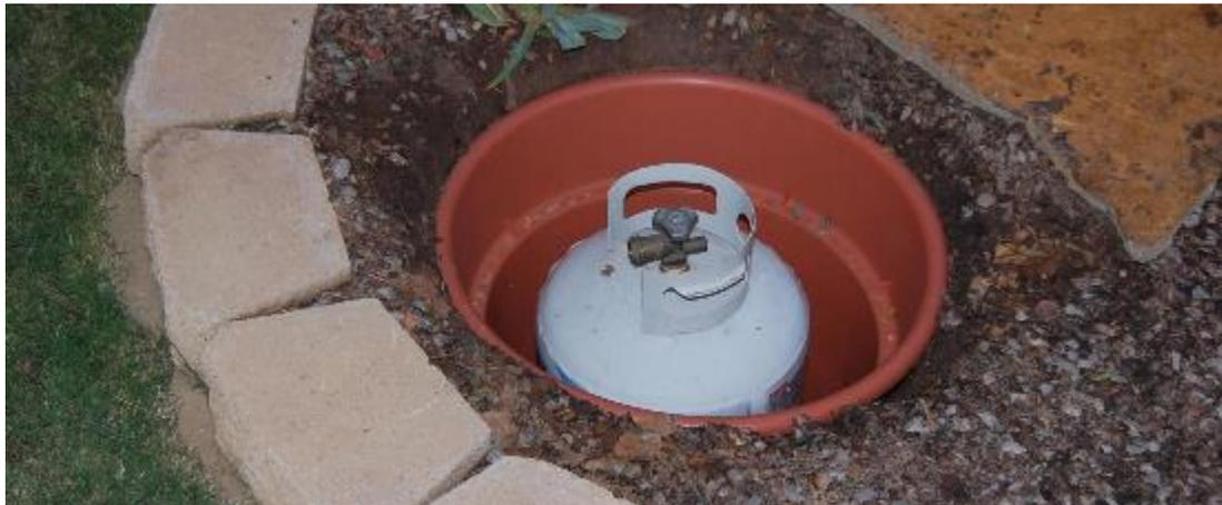
Step 7 → A form (plastic border for flowerbeds) was put around the inner circle of the fire pit to hold in the concrete. 4 bags of Quikrete were used, it dried over night and then the form was broken free.
