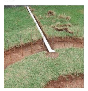
Step  $5 \rightarrow$  I decided to create a concrete base for under my Gas ring so I extended out the PVC pipe to reach to the Pit, and then I put in another drain.
