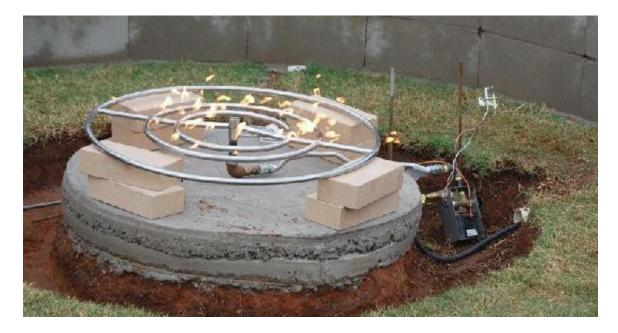
Step  $13 \rightarrow$  The footing for the fire brick and stone was poured and then the fire brick were put in. First a row of horizontal bricks and then the soldiers (vertical brick) were put into place to form a circle.
