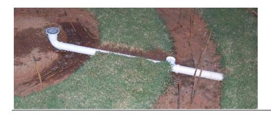
Step  $6 \rightarrow$  Running the Natural Gas line from the house to the pit was very expensive so I decided to go the propane route. I dug a deep hole in one of the adjacent flowerbeds, placed a plastic pot in it and then put in the propane tank. One piece of flagstone will be laid on top to conceal the tank.
