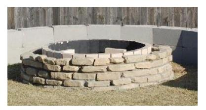
Step  $15 \rightarrow I$  finished the stone work and then poured mortar in between the fire brick and the stone for extra stability. Then I laid out the flagstone in the yard and tried to piece together this very difficult puzzle. Getting them to fit, in a circular pattern was not easy and it took about 2 hours to get a design that I was comfortable with. Once complete, I topped off the pit with more lava rock and then cleaned the stone and flagstone.
