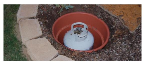
Step  $7 \rightarrow$  A form (plastic border for flowerbeds) was put around the inner circle of the fire pit to hold in the concrete. 4 bags of Quickrete were used, it dried over night and then the form was broken free.
